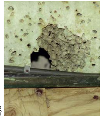
Fig.68.40, 68.41, 68.42 & 68.43: Alphitobius diaperinus (larvae). Darkling beetles are found in all kinds of structures, but more often in the walls. Larvae can drill holes in polystyrene foam, in fiberglass and insulation panels.
