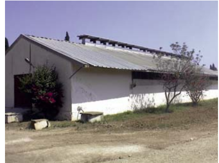
Fig.7.12: Closed building with mechanical ventilation.
