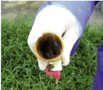
Fig.81.27: Iron clogged in water line.
