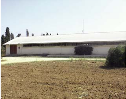
Fig.7.11: Closed building with natural ventilation.
