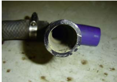
Fig.81.12 & 81.13: The biofilm layer must be peeled off from the drinking system.
